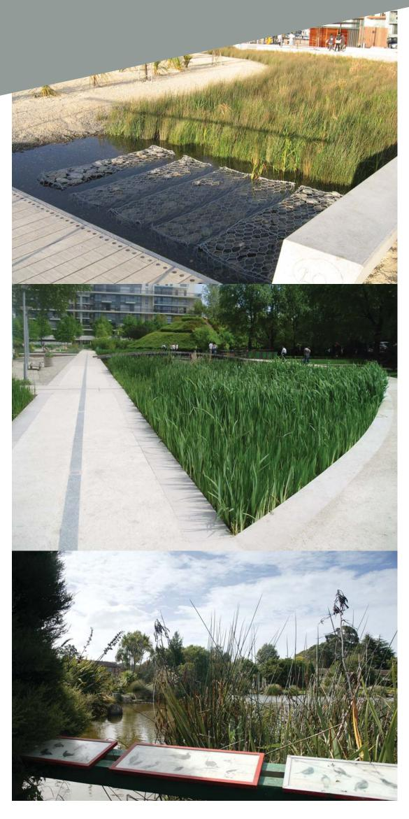
Stormwater can be treated by using planting (reeds) to filter out contaminants effectively.
